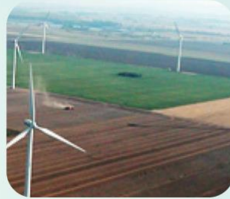
WÖRBZIG GERMANY 30 MW
